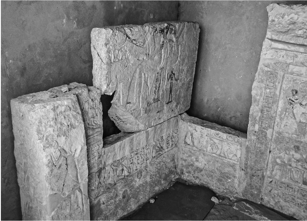
Figure 8. Chapel of Tatia after reinstallation of the slab on the south wall.
