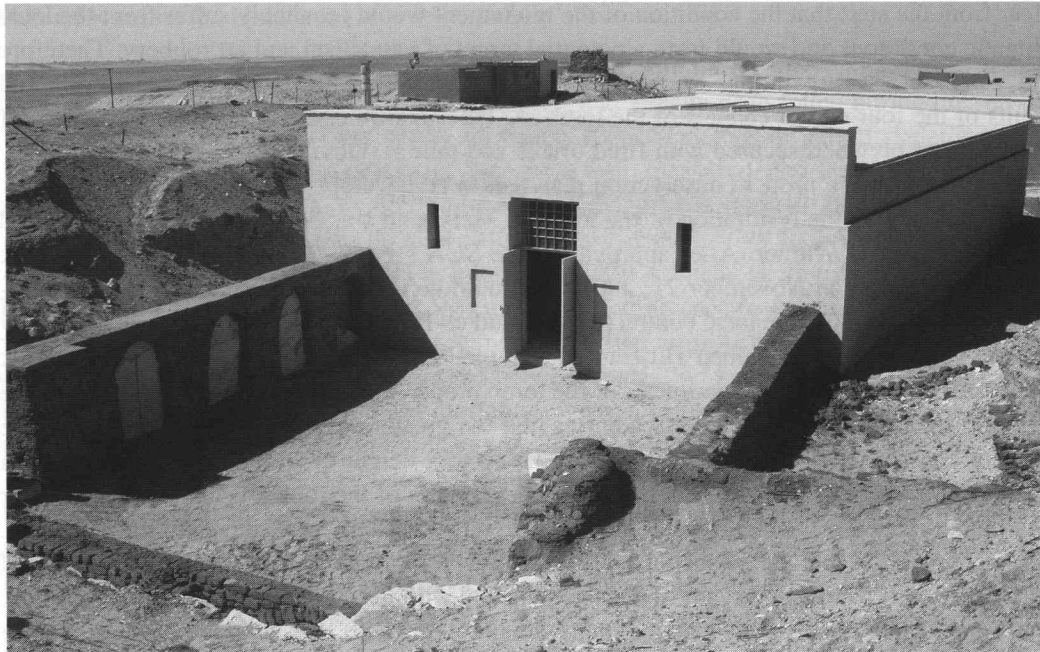
Fig. 9. Exterior view of the shelter constructed over the tomb of Meryneith.
